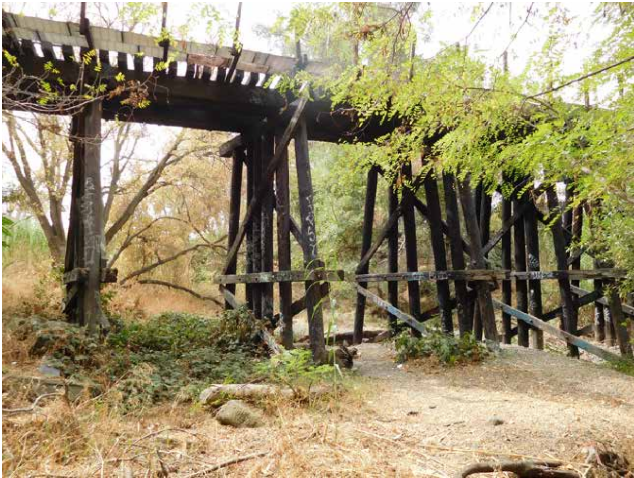
Photo 1: CA_Santa Clara County_Willow Glen Trestle_0001.tif
