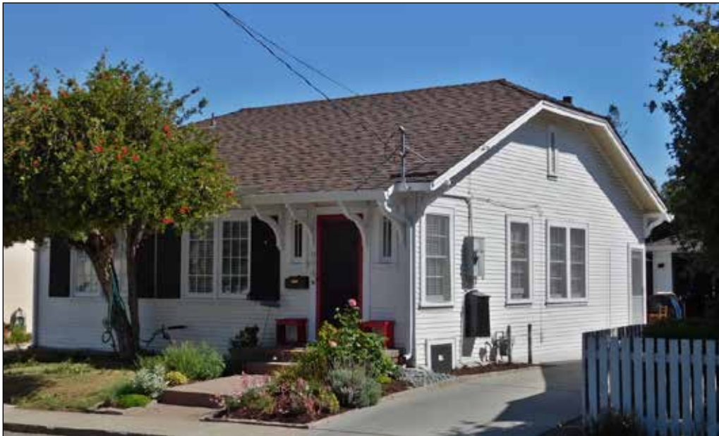
Figures 5 and 6. Two images of extant historic homes lining Ramona Court and financed by T.S. Montgomery's Standard Realty Company. Top: 990 Ramona Court. Bottom: 994 Ramona Court.
