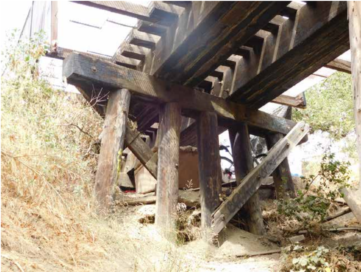
Photo 6: CA_Santa Clara County_Willow Glen Trestle_0006.tif
