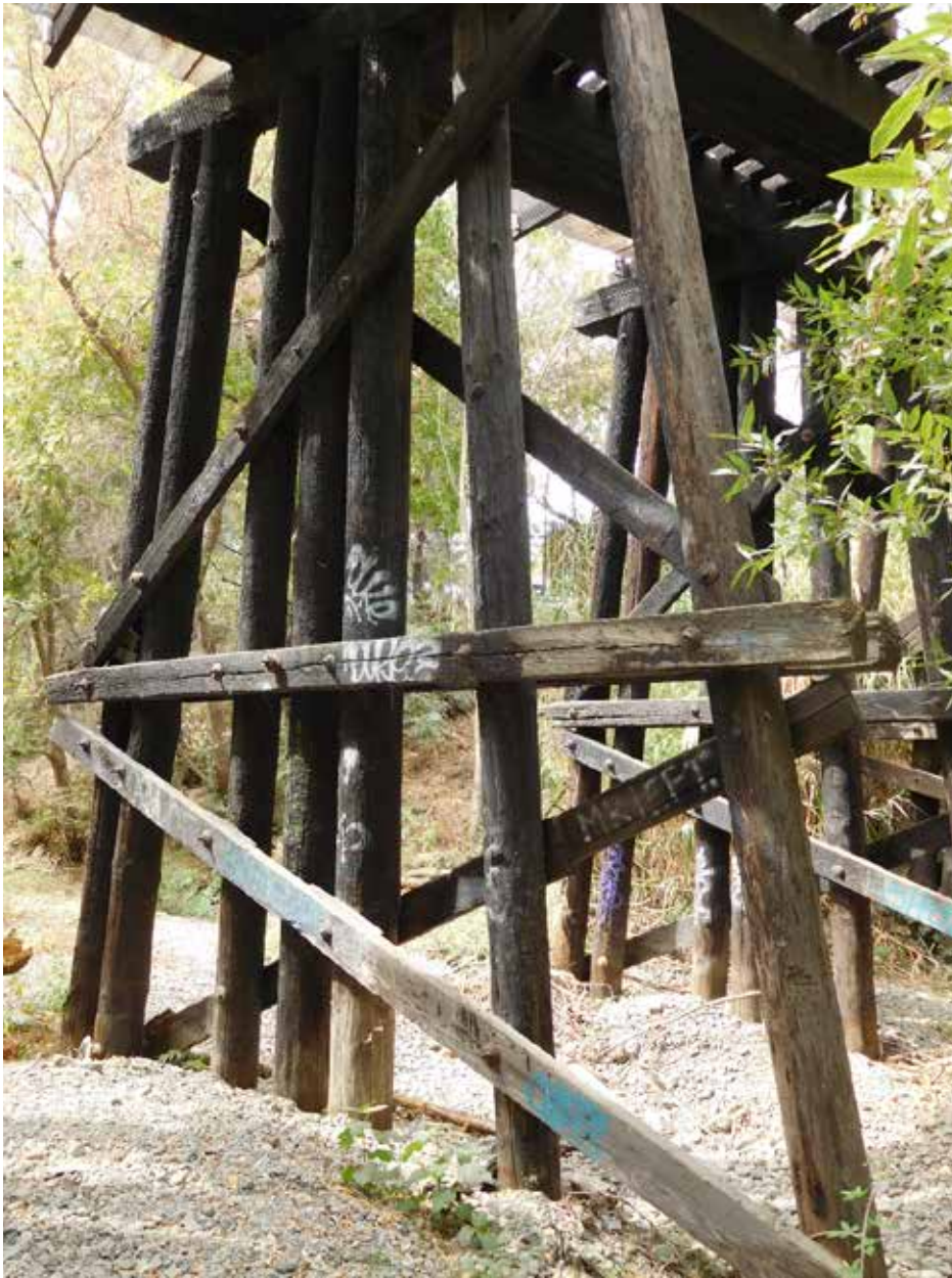
Photo 10: CA_Santa Clara County_Willow Glen Trestle_0010.tif
