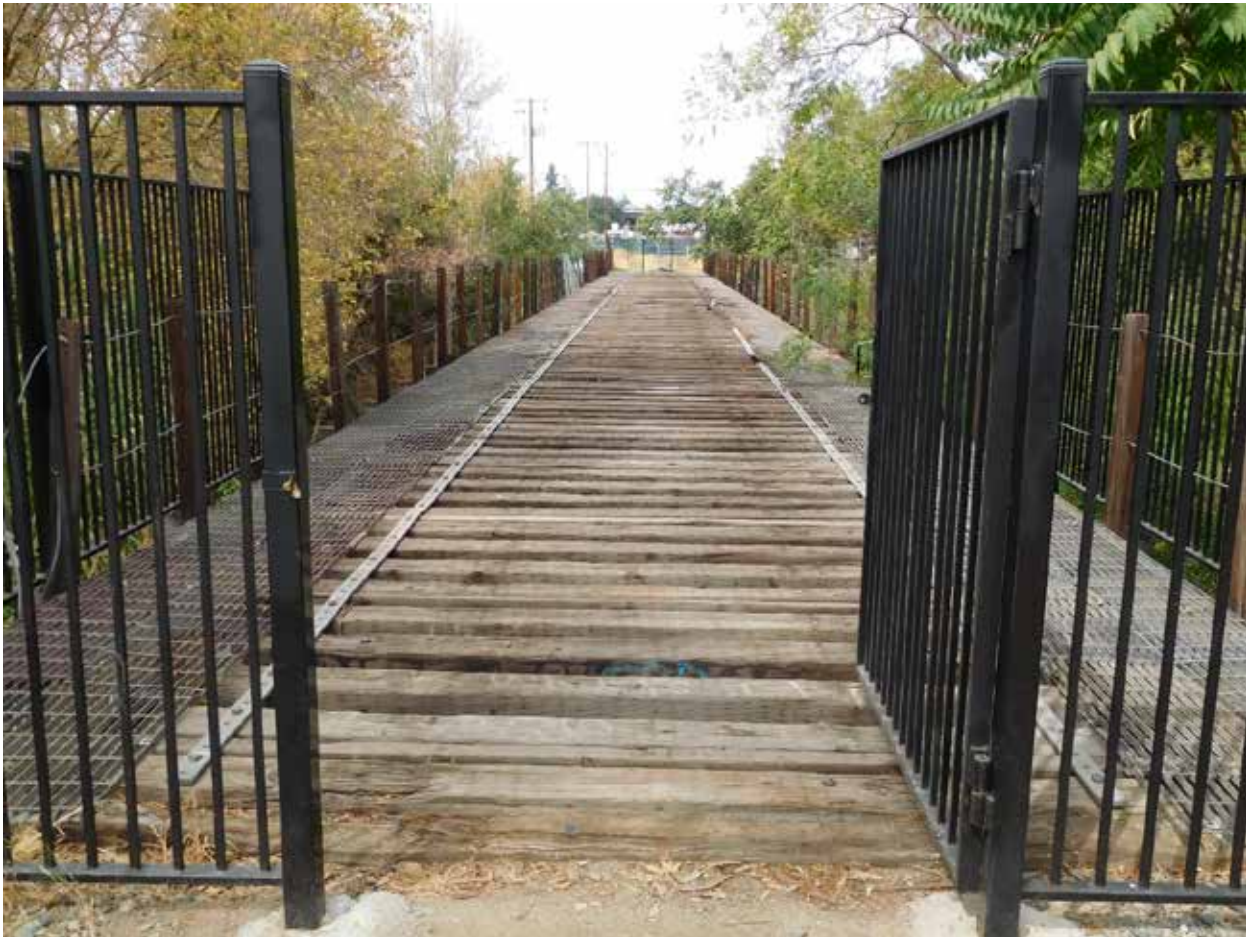
Photo 5: CA_Santa Clara County_Willow Glen Trestle_0005.tif
