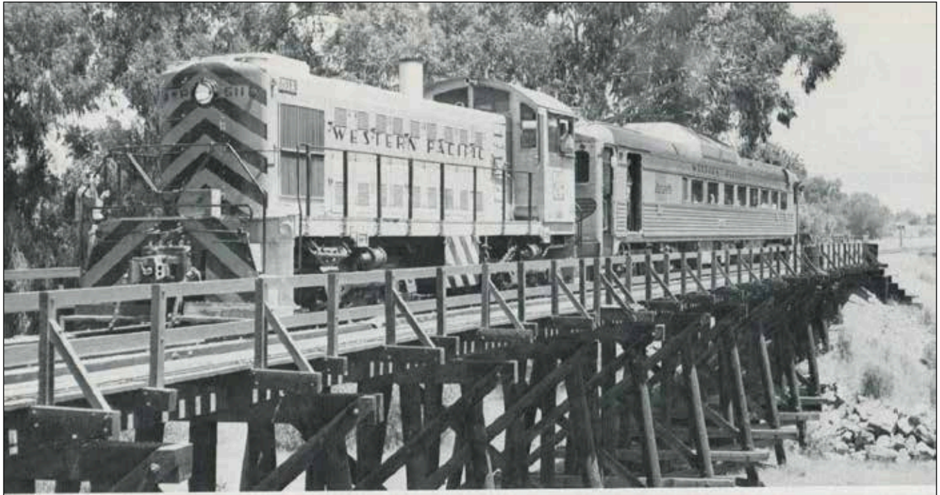
Figure 2. Willow Glen Trestle looking northwest, showing a train crossing the bridge, in 1955 (Courtesy: Norman Holmes, Prune Country Railroading , Shade Tree Books, 1985).
