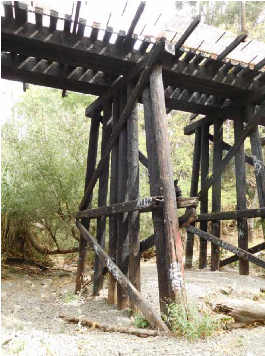
Photo 11: CA_Santa Clara County_Willow Glen Trestle_0011.tif
