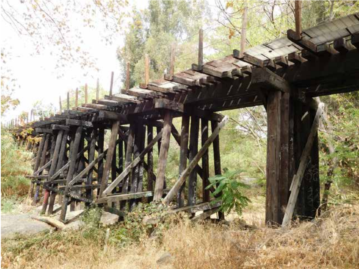
Photo 2: CA_Santa Clara County_Willow Glen Trestle_0002.tif
