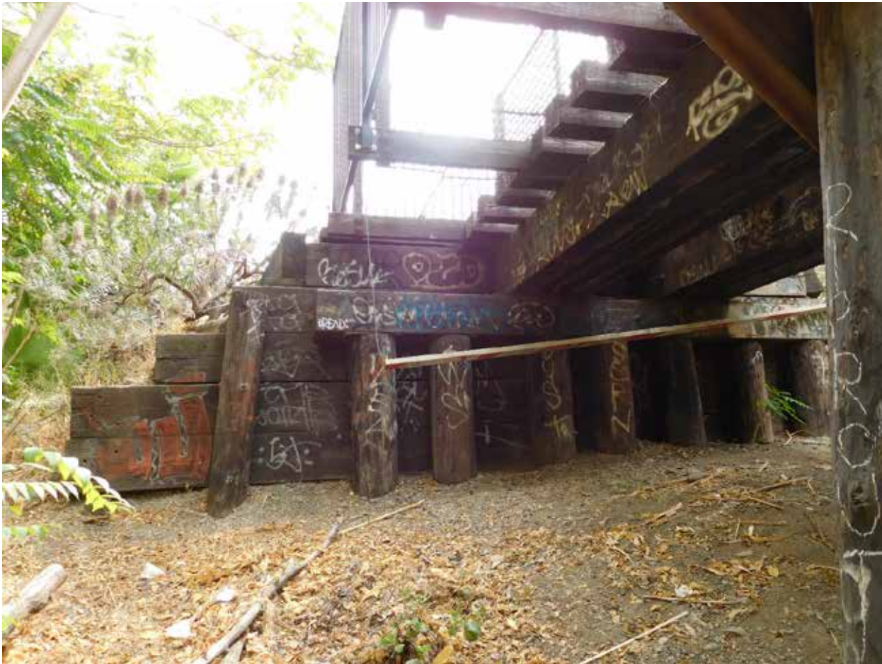
Photo 8: CA_Santa Clara County_Willow Glen Trestle_0008.tif
