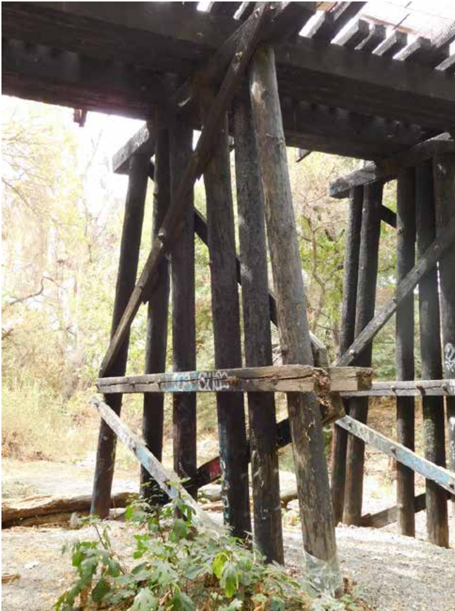
Photo 9: CA_Santa Clara County_Willow Glen Trestle_0009.tif
